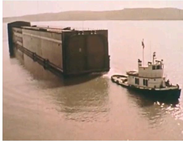
63rd Street Tunnel Section Pulled by Tugboat
